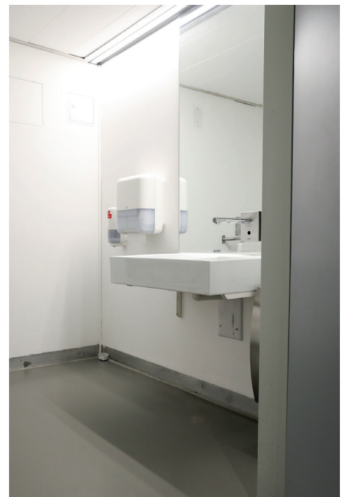
Barrier-free WC in the basement
