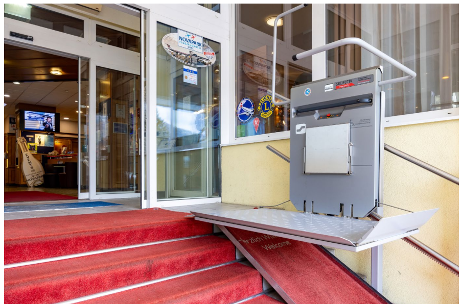
Entrance with stair lift
